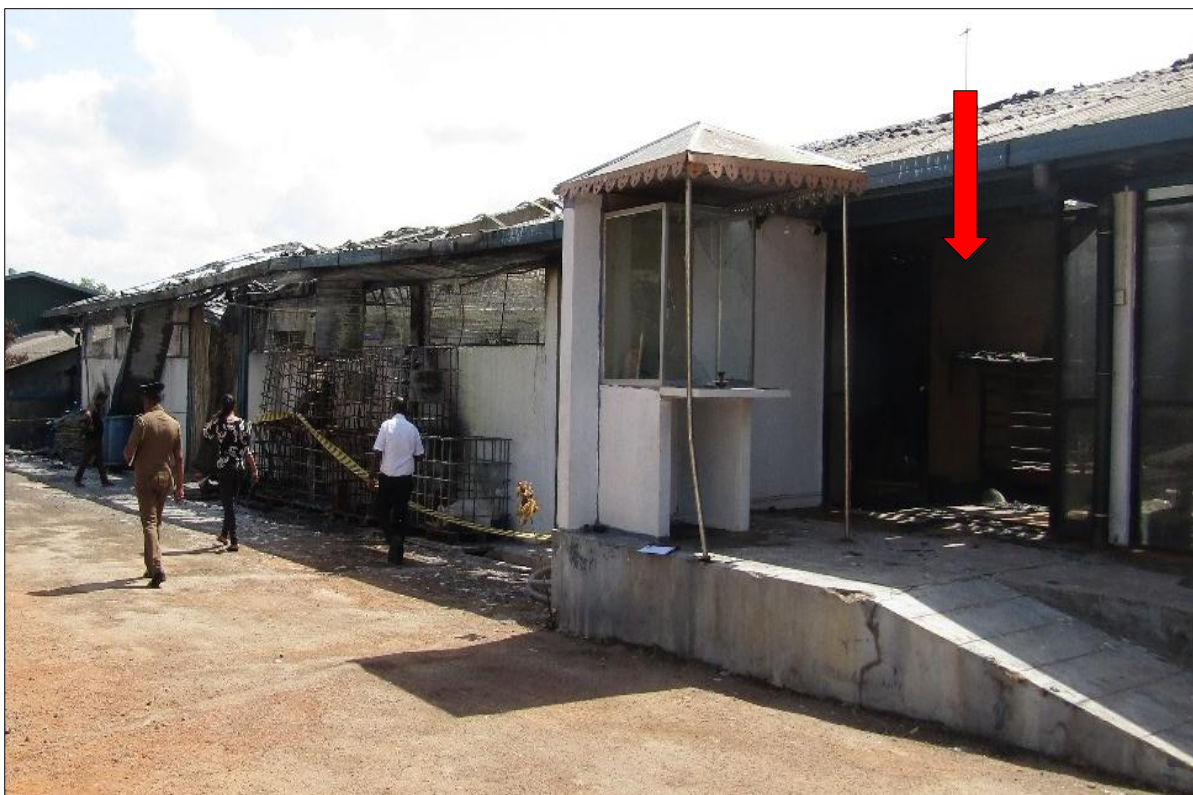
Figure 1: Outer view of the burnt warehouse, built attached to the office part (slightly damaged front office part indicated by the red arrow)
