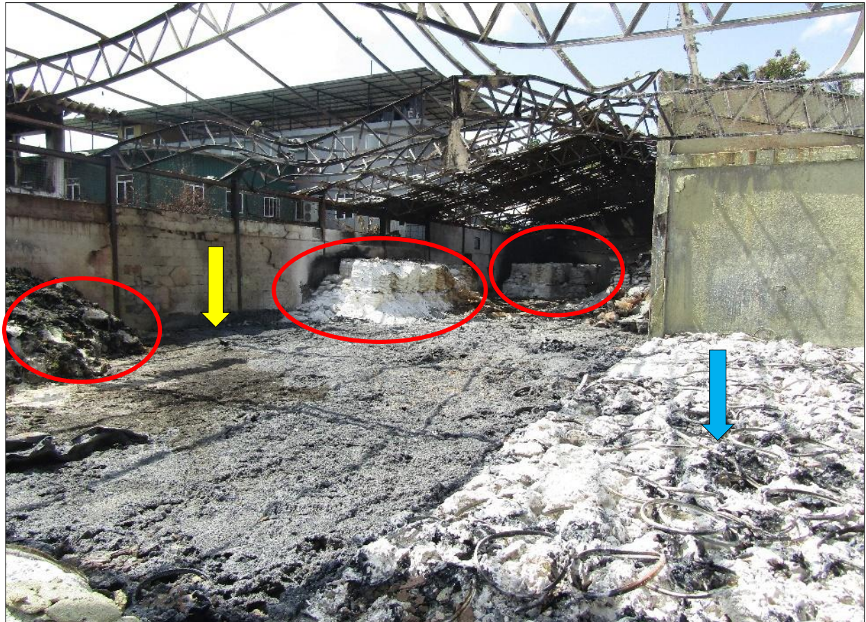
Figure 4: Sites where sodium carbonate packages were stacked (red circles) and the intensely burnt area (yellow arrow), site where the 35% calcium hypochlorite was stacked (blue arrow).
