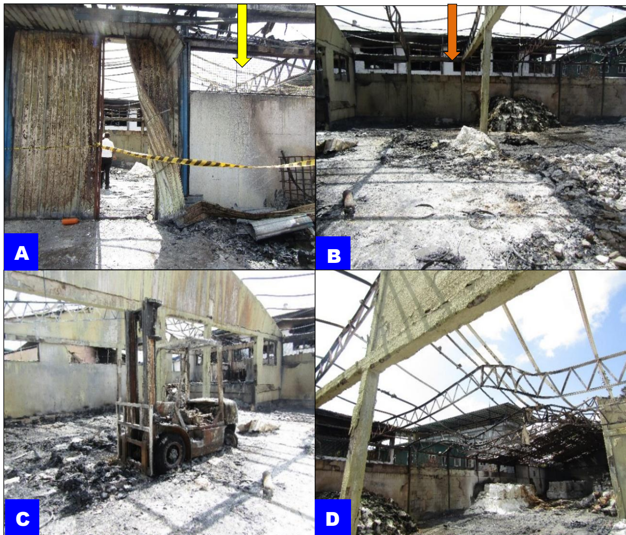
Figure 2: Close-up structural views of the burnt warehouse: (A) Main entrance door forced-open by the firefighters and metallic grill structure on the front wall (yellow arrow); (B) Inner view opposite the main entrance and metallic grill structure on the back wall (orange arrow); (C) Burnt forklift machine kept at the left front side; (D) Severely damaged inner structure in the right direction.
